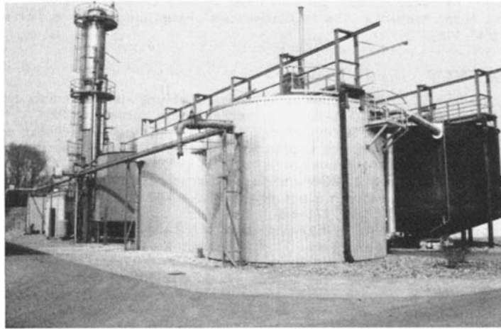
Fig 7: ATS facility for 80,000 P.E. (Niersverband; sludge throughput 75 \text{ m}^3/\text{d} ; reactor volume: 2 \times 180 \text{ m}^3 ; in operation since 1981) the thermal pasteurization unit in the background left was replaced by the ATS
